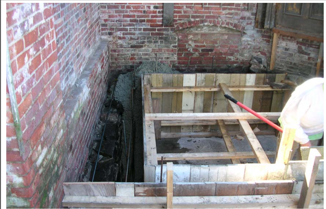
Tower Wall: Concrete Placement in progress.
