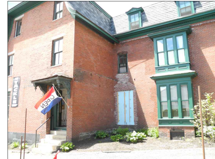
AREA OF WORK AND EXISTING ADJACENT PORCH
