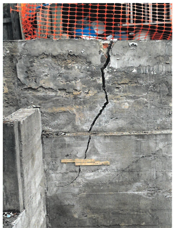
Picture 4: Large Crack in Retaining Wall
