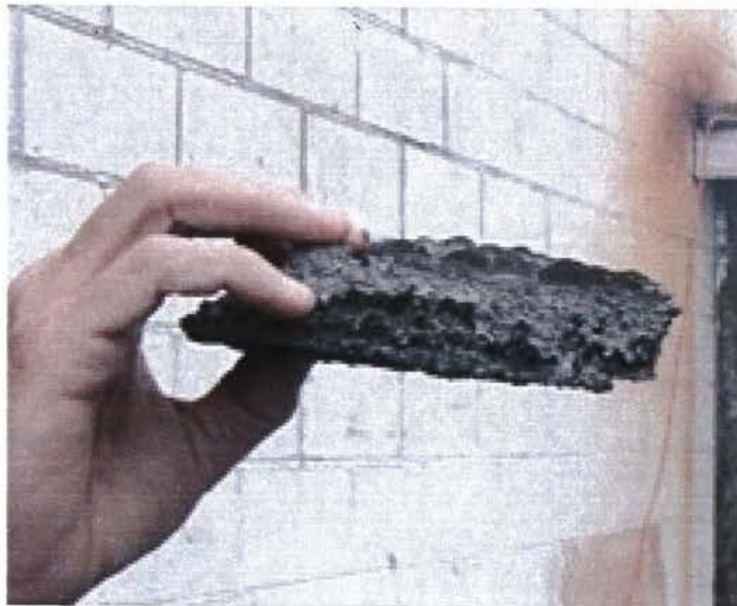
Illustrating thickness of intumesced coating
