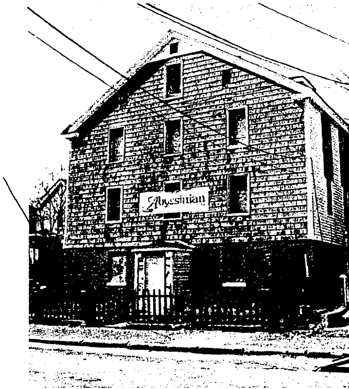
Photo 7: Exterior view looking W
