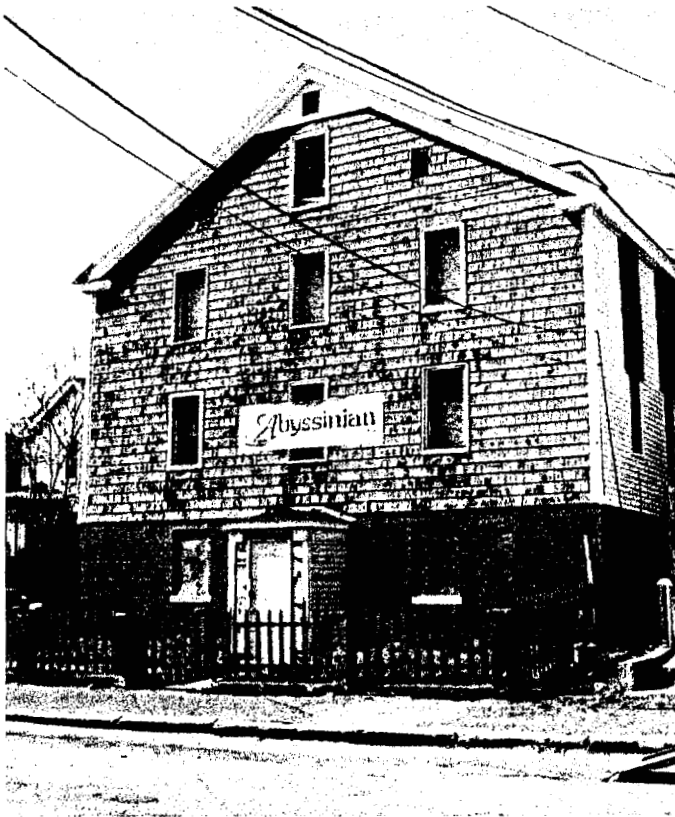
Photo 7: Exterior view looking W
