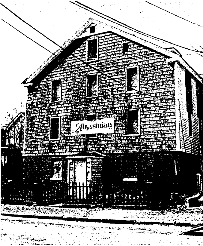
Photo 7: Exterior view looking W
