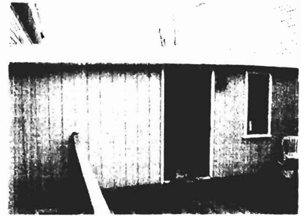
Storage at rear of 65 Newbury Street
