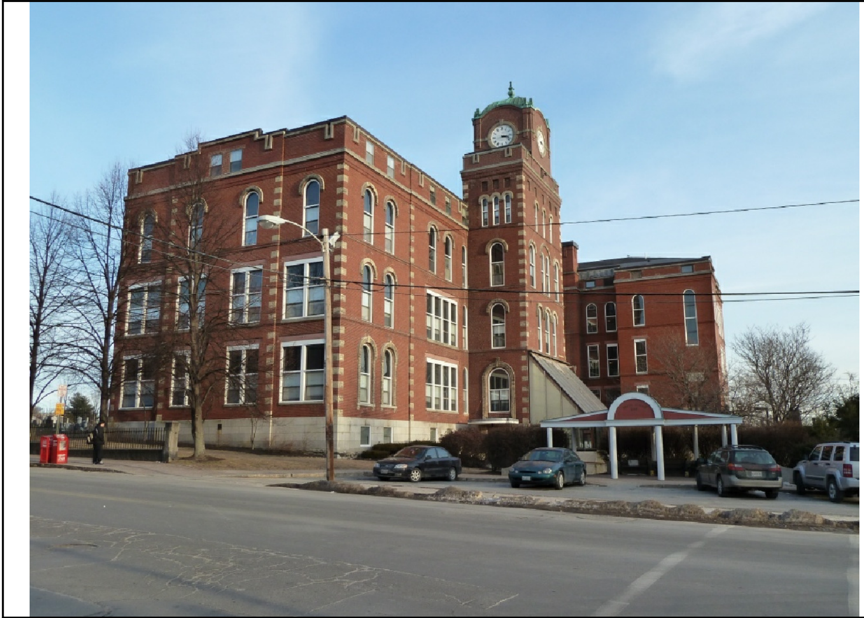
H14 SITE PHOTO #2 NO SCALE
