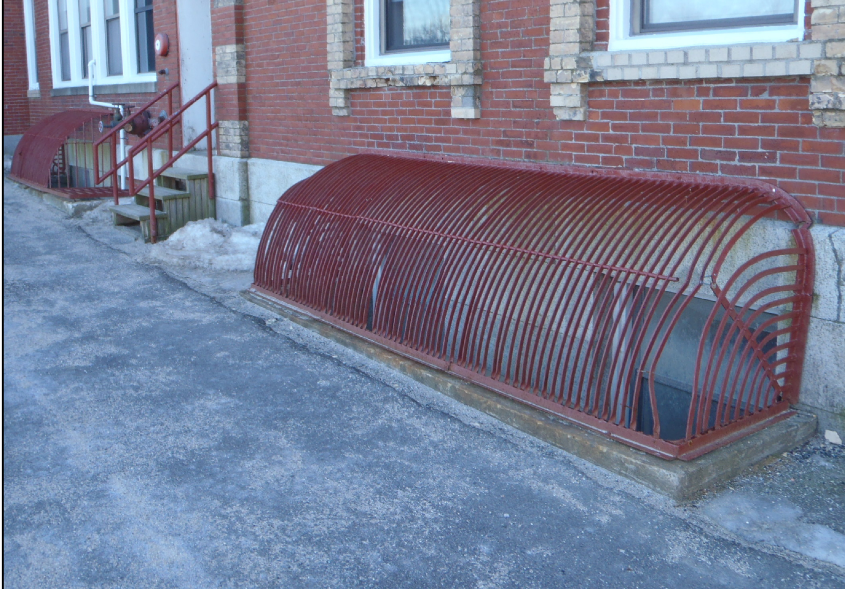
D14 SITE PHOTO #3 NO SCALE
