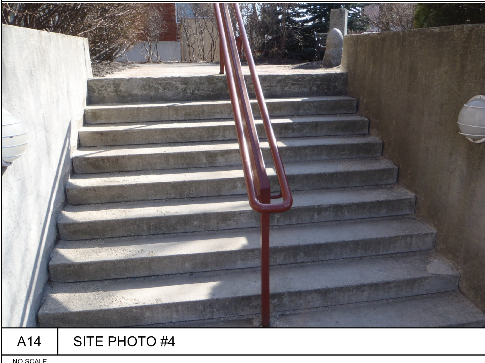
A14 SITE PHOTO #4 NO SCALE
