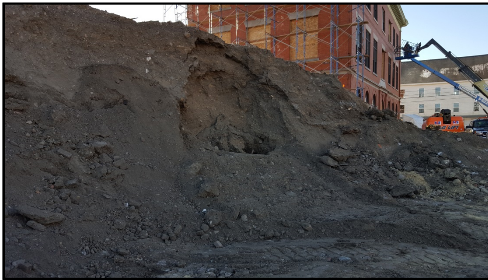
Photo 1: Stockpile within proposed building footprint, December 2016
