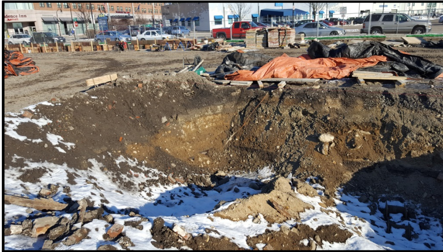
Photo 2: Foundation excavation for hotel directly east of the proposed building footprint
