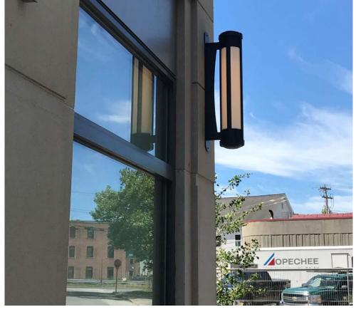
Our proposed sconce is Nighttime Friendly which reduces any negative impacts on the nighttime environment. Products typically selected as Nighttime Friendly have no uplight, meet the IESNA definition for full cutoff optics and reduce high-angle brightness. These measures of luminaire performance are consistent with sustainability standards for light pollution reduction.
