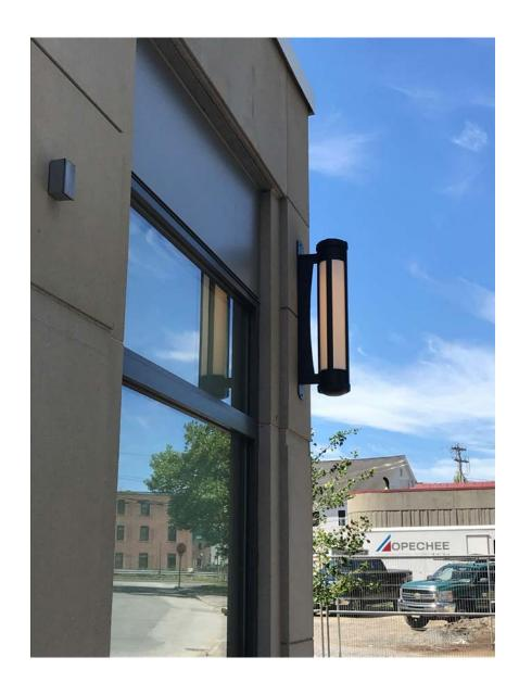
We selected this sconce to be Nighttime Friendly, which attempts to minimize the impact of electric lighting systems onto the nighttime environment. Focus is on reduction of light pollution.
