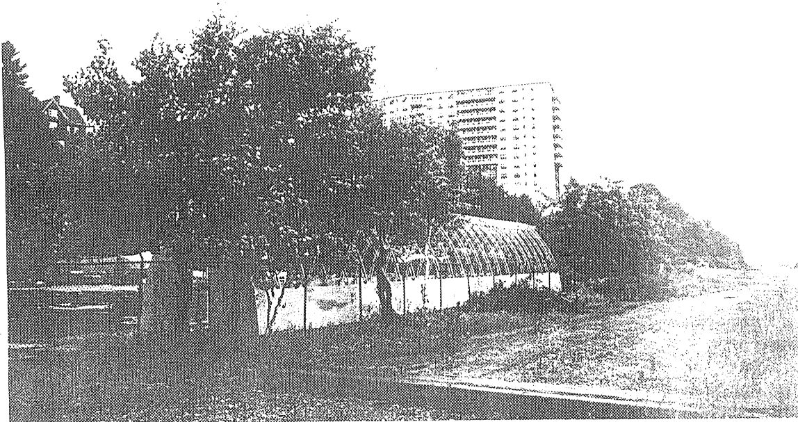
ENGINE SHELTER LOOKING NORTH
