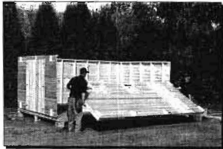
Your new shed is complete in just a few hours!
