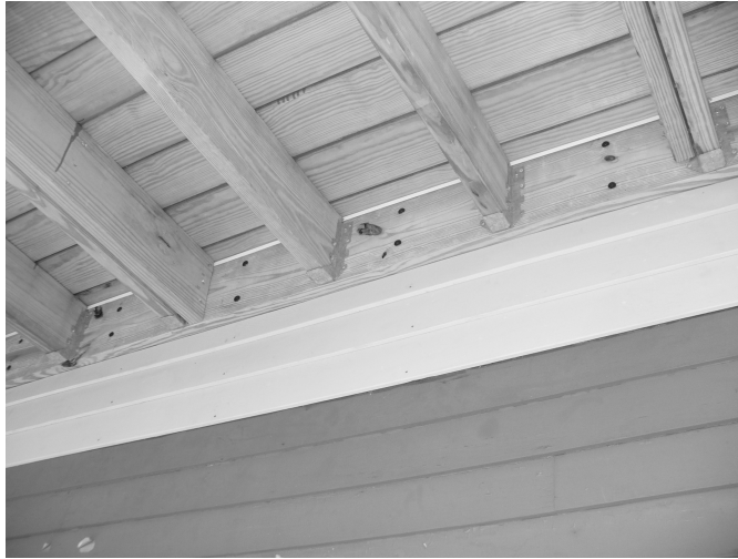
Scope 1.2.1.2 - attach (3) decks to house at ledger.
