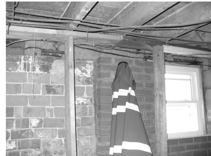
Existing Conditions at Floor Joists
