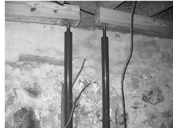
Existing Conditions at Floor Joists
