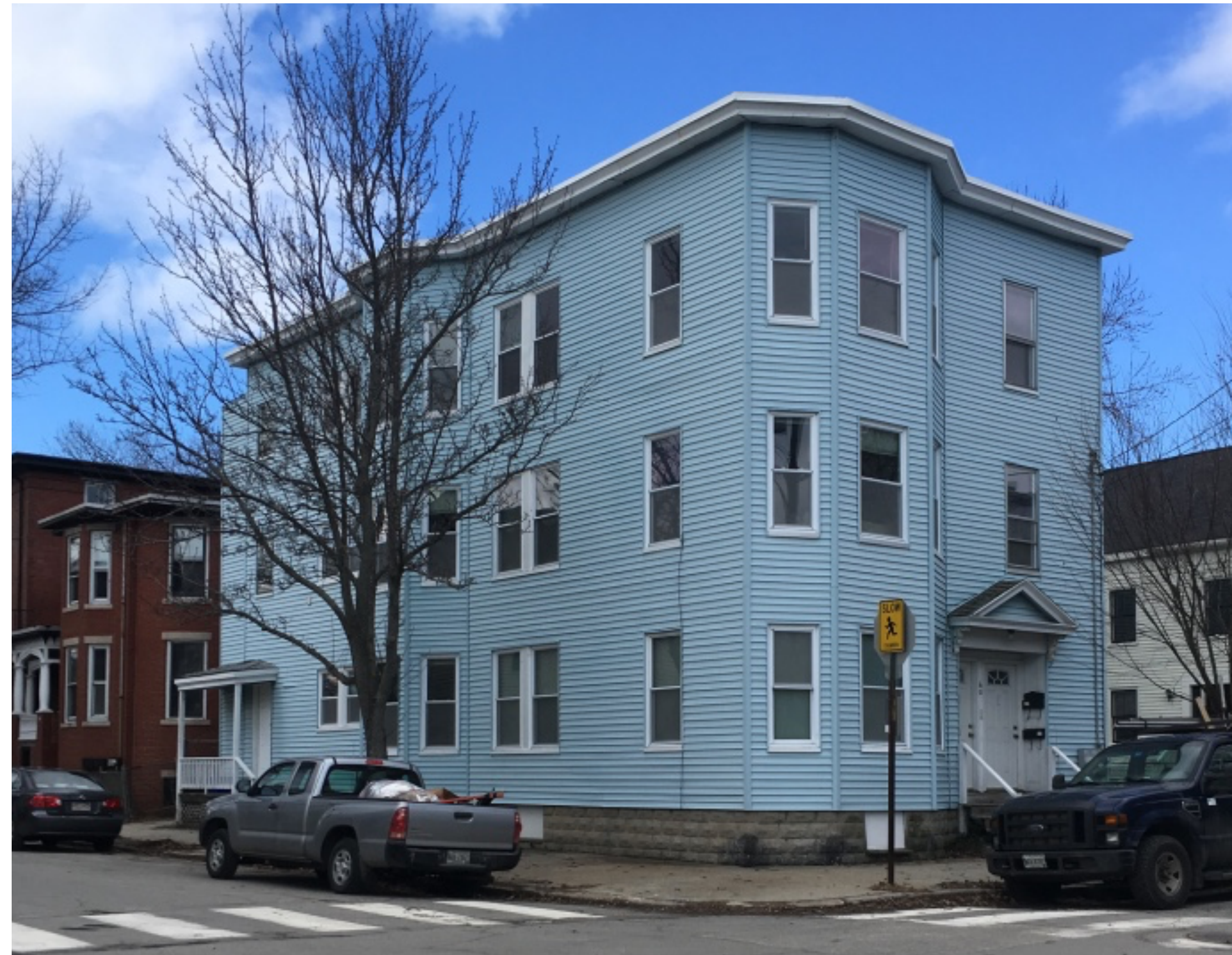
1 EXISTING CORNER VIEW SCALE: 1:0.83
