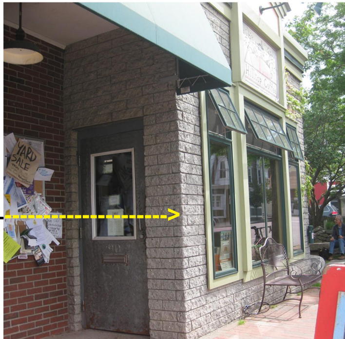
detail of existing vestibule; proposed vestibule doors & side panels to align with building face----->
