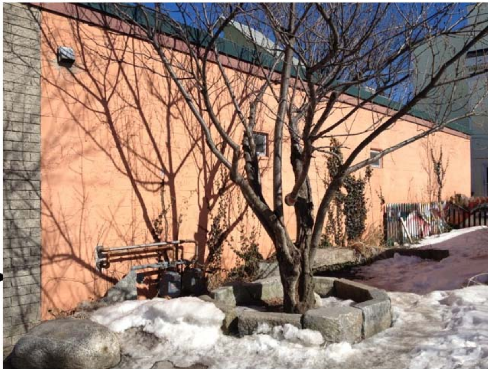
Side Wall Facade
