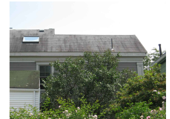
EXISTING RIGHT SIDE PHOTO
