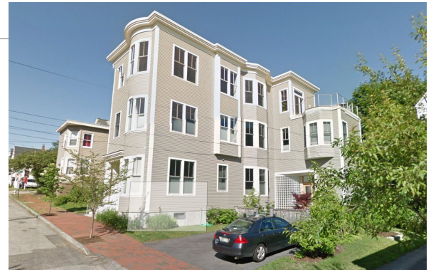
(1) 46 Turner St Multi-family flat roof structure on the project block
