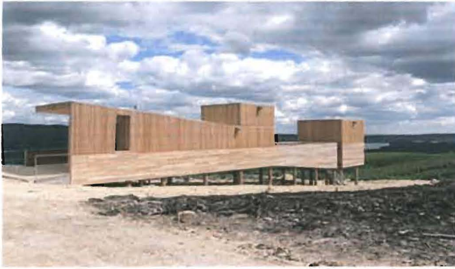
Kielder Water and Forest Park, Northumberland, UK by Charles Barclay Architects
