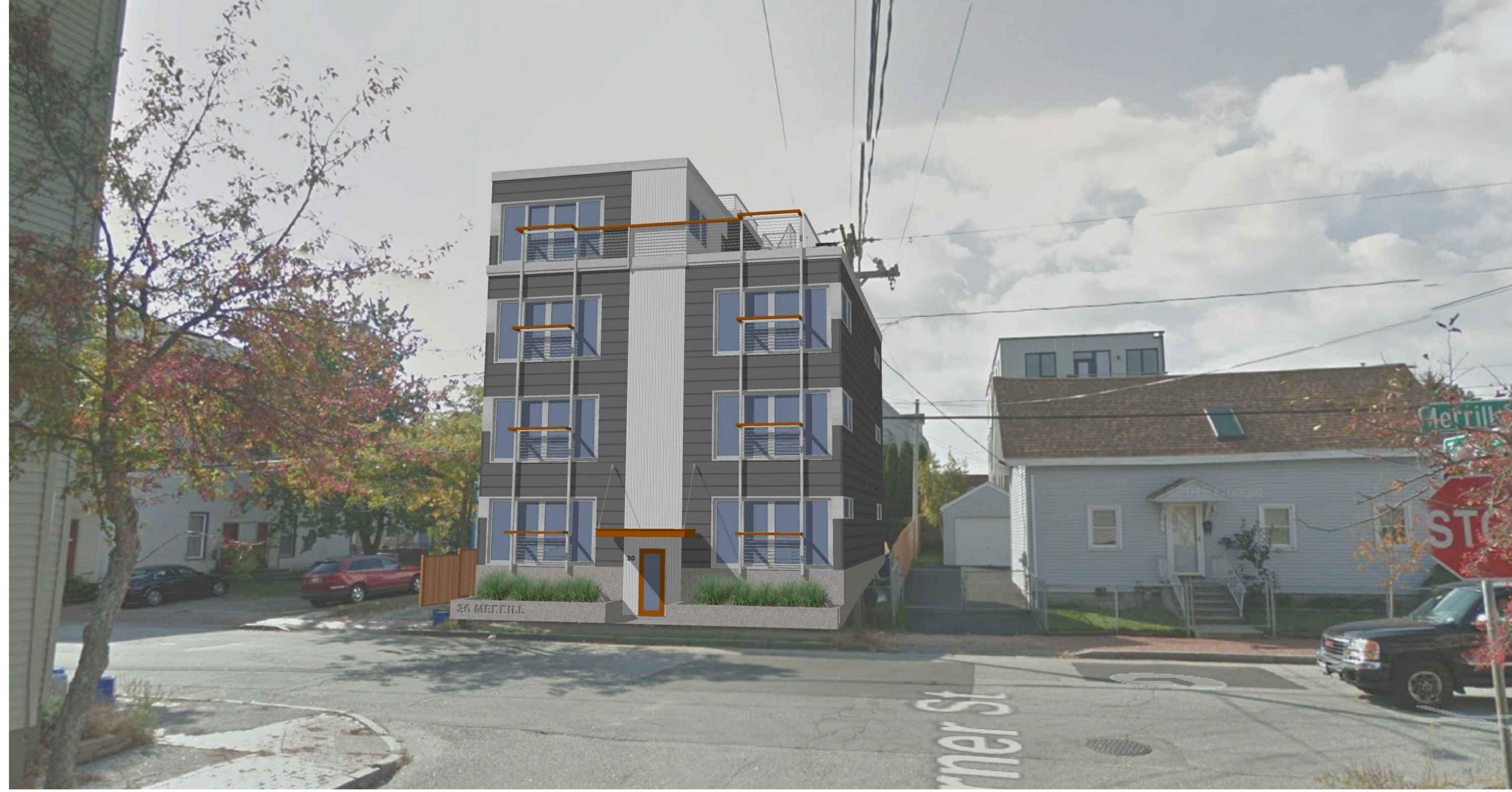
TURNER STREET VIEW
