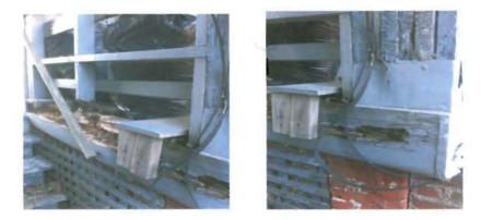
2<sup>nd</sup> floor deck framing: Replace rotted support wood as needed.
