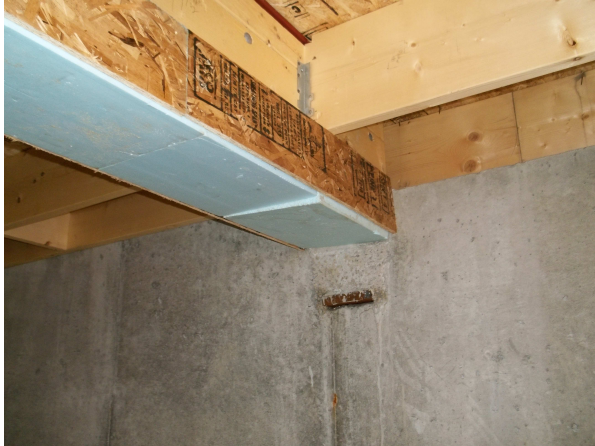
Photo # 1 – Steel beam Pocket filled w/ concrete
