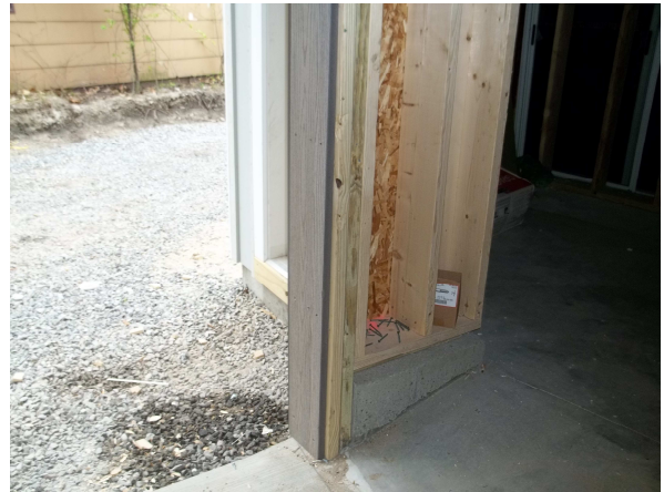
Photo #2 – Pressure treated jack studs at doors
