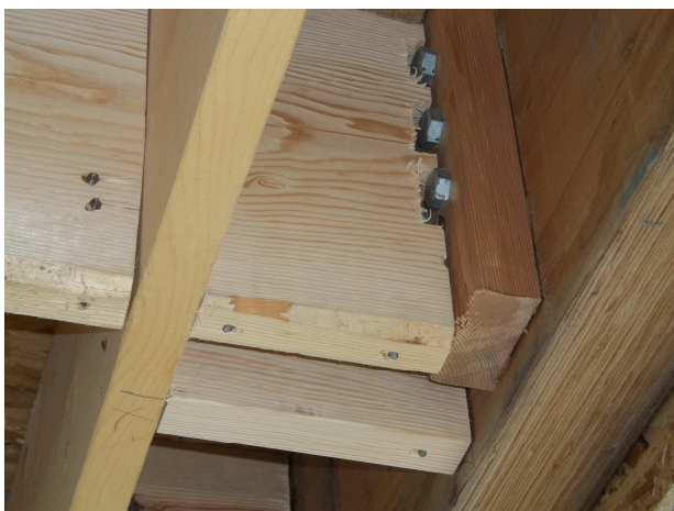
Photo # 11 – Guardrail post base reinforcement
