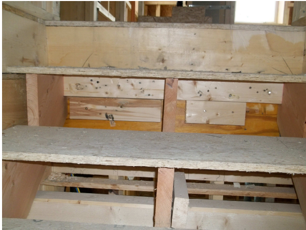
Photo # 7 –Ledger added below stringer- top stair
