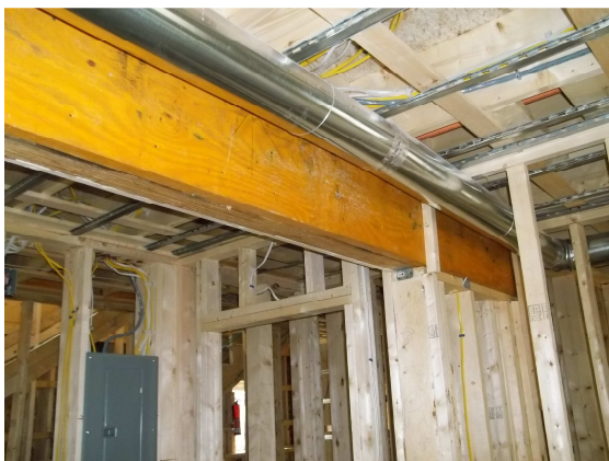
Photo # 5 –VLAM sister added @ 1 st floor beam
