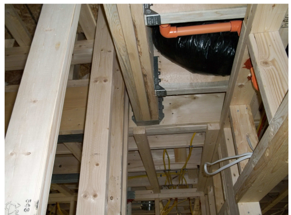
Photo #6 – Beam Hangers added near elevator
