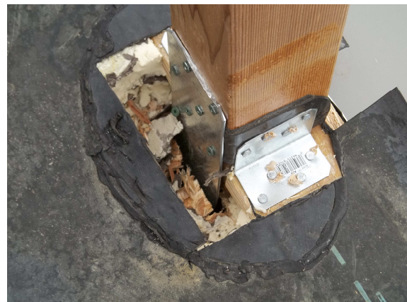
Photo #10 – Guardrail post base reinforcement
