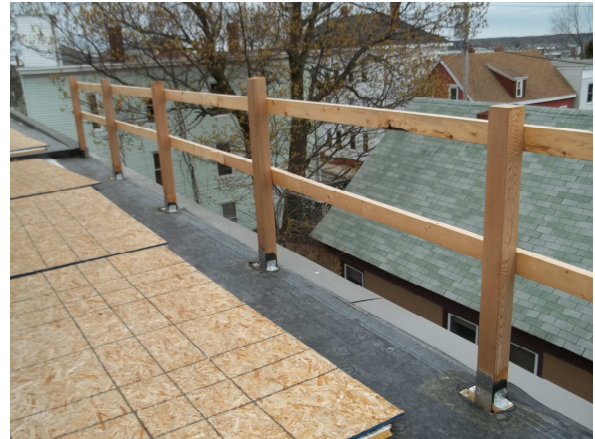
Photo #8 – Guardrail post base reinforcement
