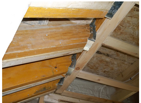
Photo #4 – Stair stringer supports
