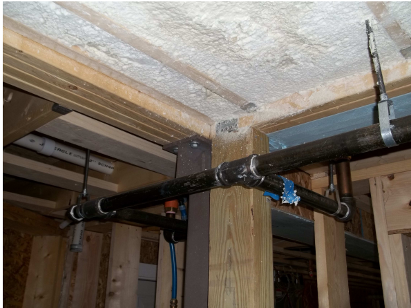
Photo # 3 – Post supporting 1 st floor beam
