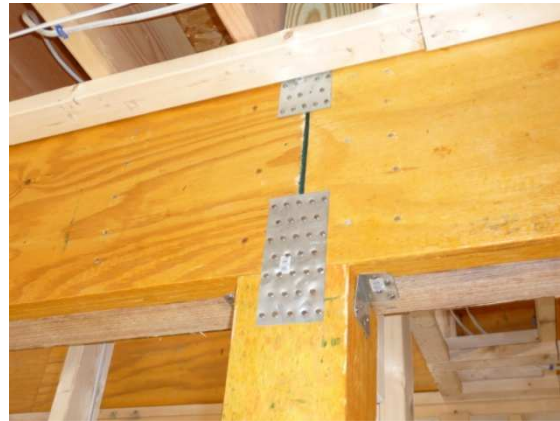
Photo #18 – 2 nd Flr: Beam to column connection
