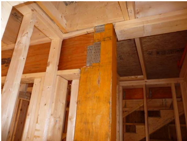
Photo # 9 – 1 st Flr: Spliced column replaced correctly
