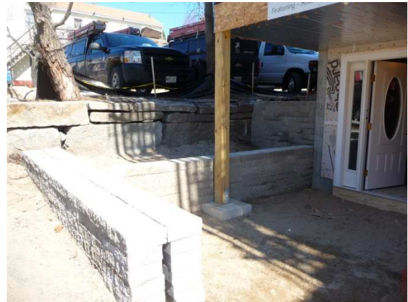
Photo #4 – North entrance – note post base anchor
