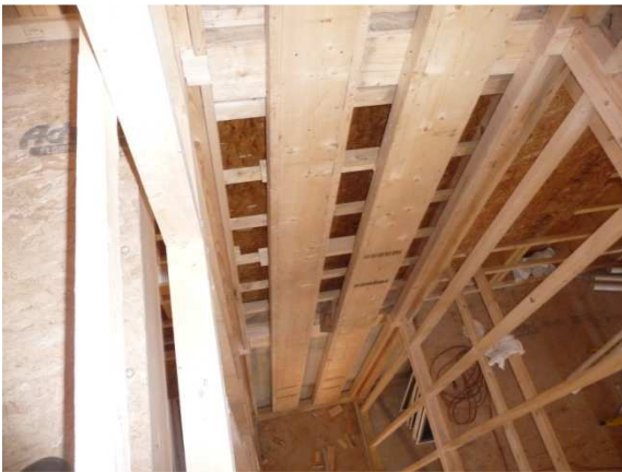
Photo # 17 – 2 nd Flr: Elevator shaft framing
