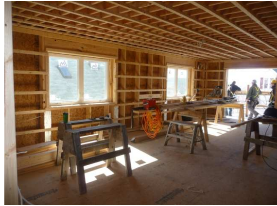
Photo #20 – 2 nd Flr: View looking north
