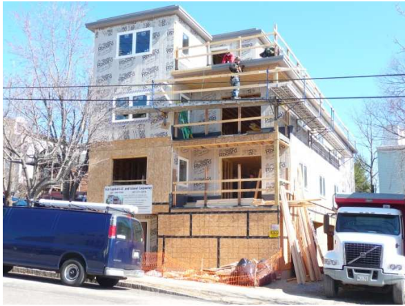
Photo # 1 – North elevation
