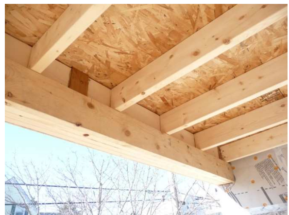
Photo #12 – 1 st Flr: Guardrail @ reduced beam
