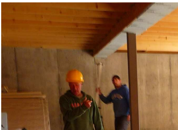
Photo # 5 – Steel beam pocket filled in with concrete
