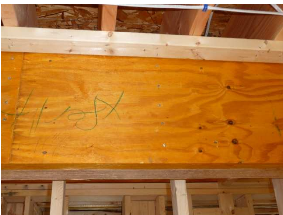
Photo # 23 – 3 rd Flr: Top loaded multi-ply beam
