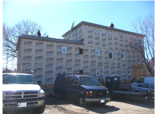
Photo #2 – East elevation
