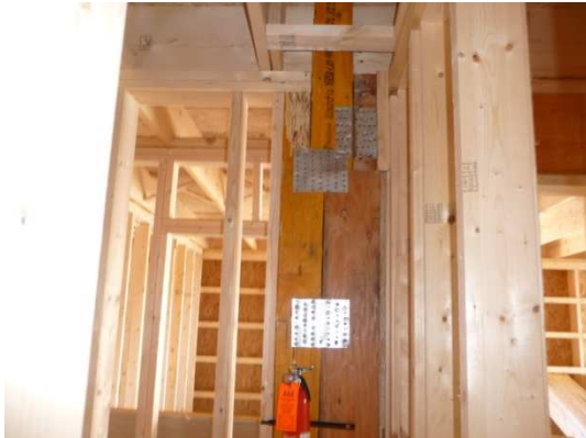
Photo # 1 – Replace spliced column
