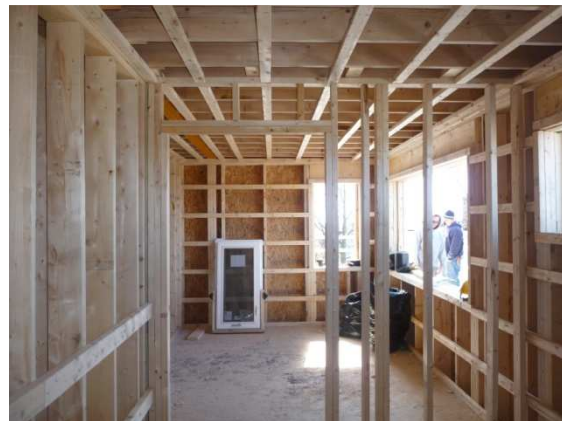
Photo #4 – Framing at top floor level
