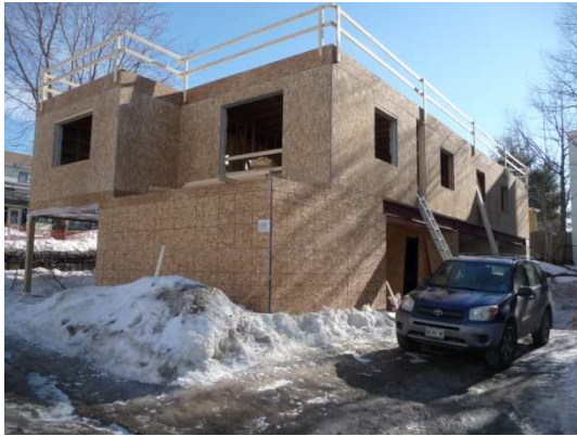
Photo # 1 – Overall View
