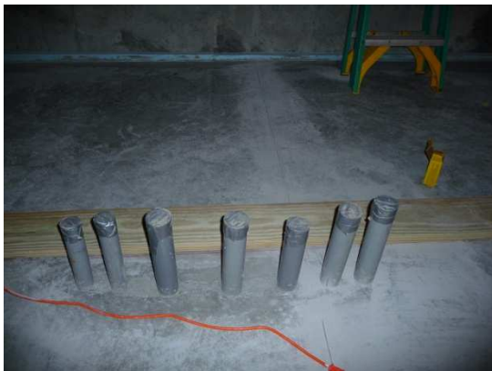
Photo # 3 – Utilities at Slab Penetrations
