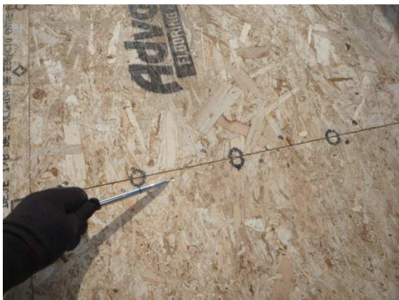
Photo # 5 – Nail spacing at floor sheathing edges
