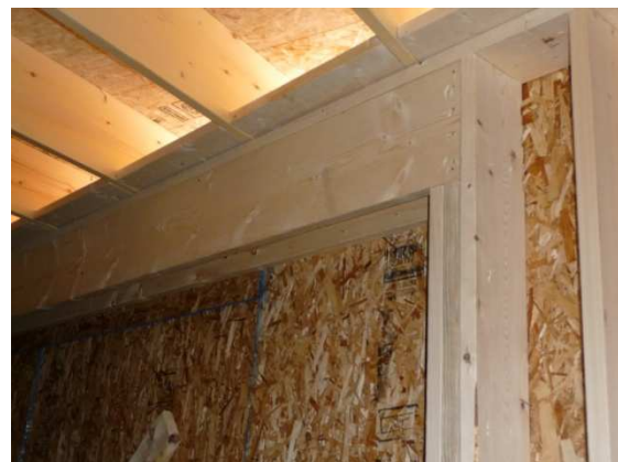
Photo #6 – Double jack studs at garage lintels
