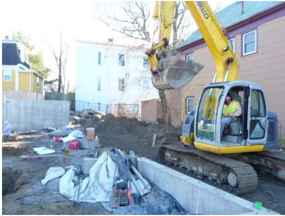
Photo # 1 – Jeff Munn Excavation
