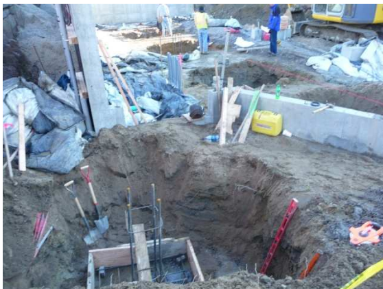
Photo # 5 – Formwork for footing at grid A/1
