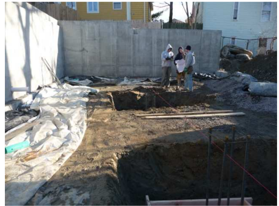
Photo #4 – Foundation wall with beam pocket
