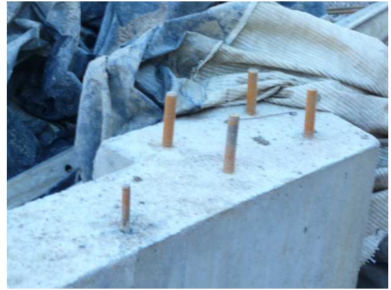
Photo #2 – Concrete pier placed previously
