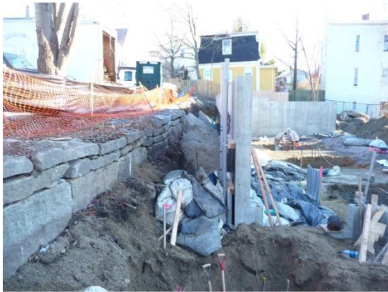
Photo # 3 – Existing retaining wall at left
