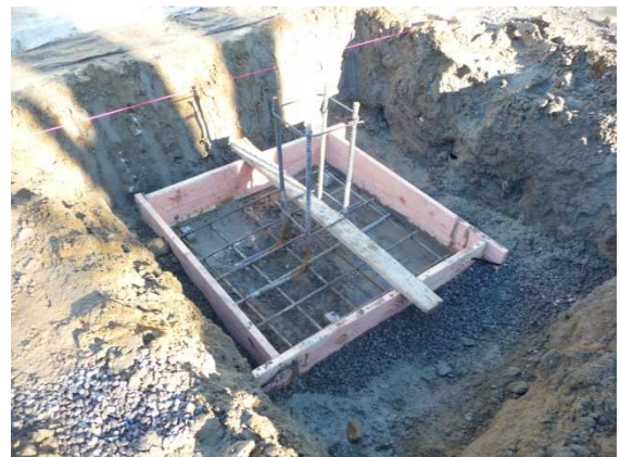
Photo #6 – Formwork for interior A.9 footing
