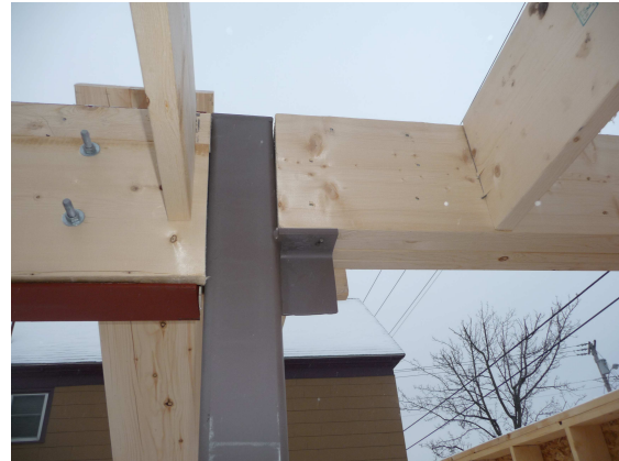
Photo #4 – Beam connection at grid 2.1/A.9
