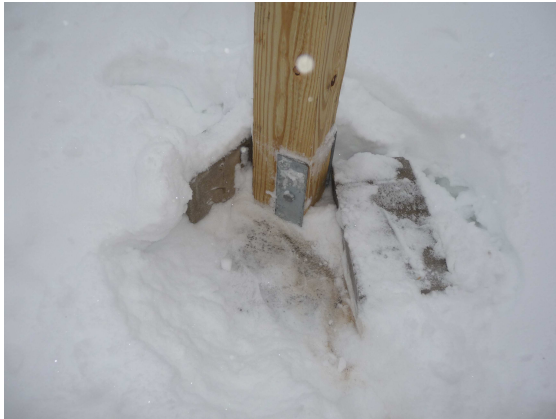
Photo # 3 – Simpson post base bracket as specified
