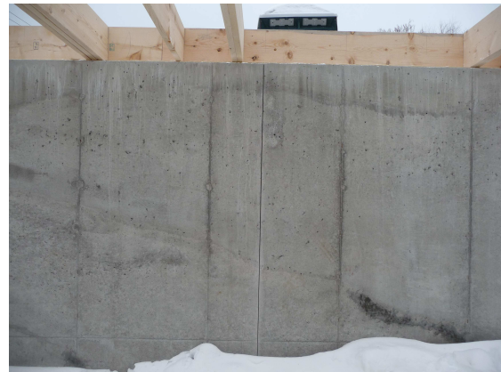
Photo #6 – Vertical concrete control joint installed
