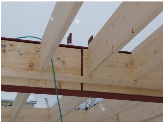
Photo # 5 – Bracket on steel beam with stiffeners below
