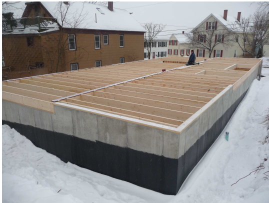
Photo # 1 – Joist installation
