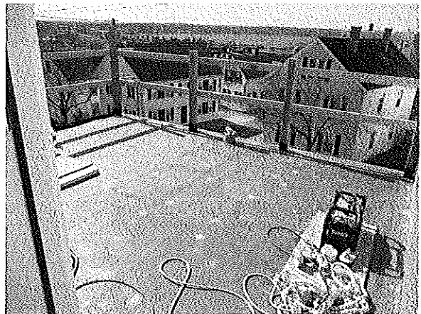
Photo #24 – 3 rd Flr: View looking at Back Cove
