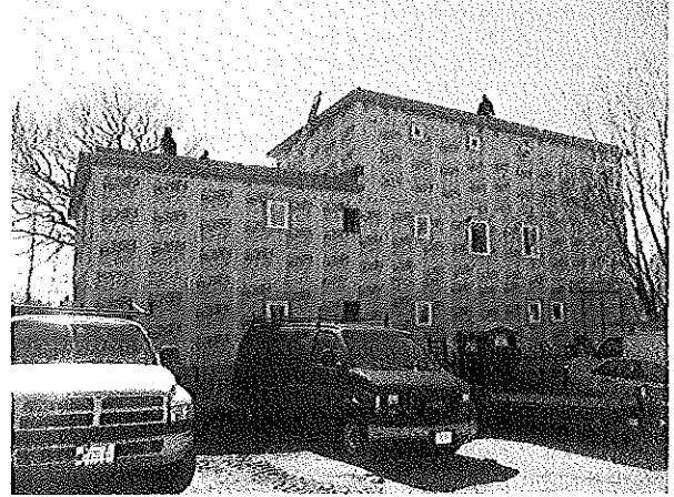
Photo #2 – East elevation
