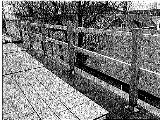
Photo #8 – Guardrail post base reinforcement
