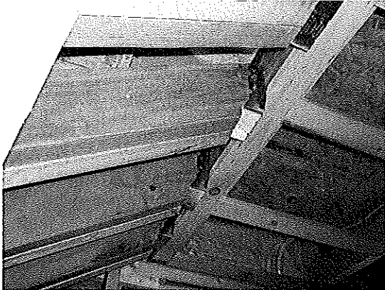
Photo #4 – Stair stringer supports
