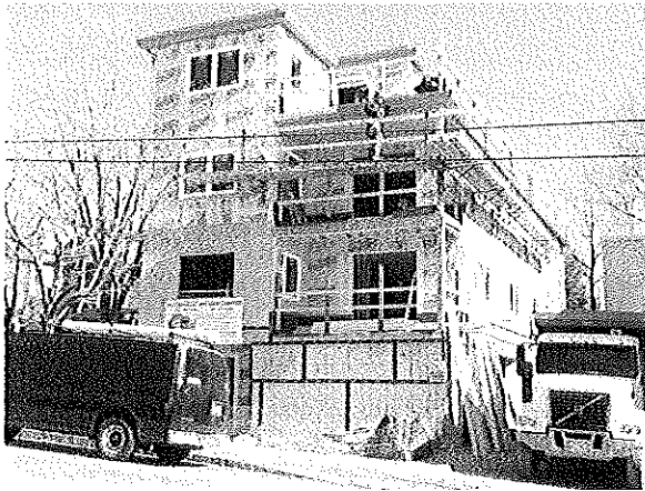
Photo # 1 – North elevation
