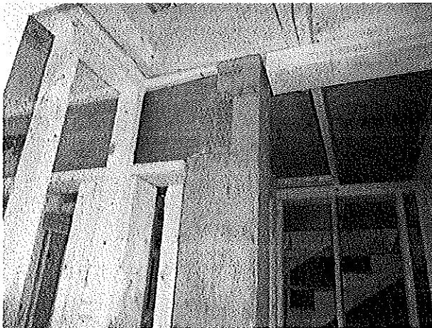
Photo # 9 – 1 st Flr: Spliced column replaced correctly
