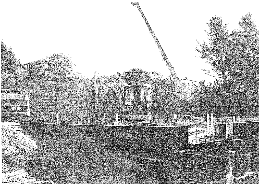
Photo 3 – Crane for steel erection shown in background
