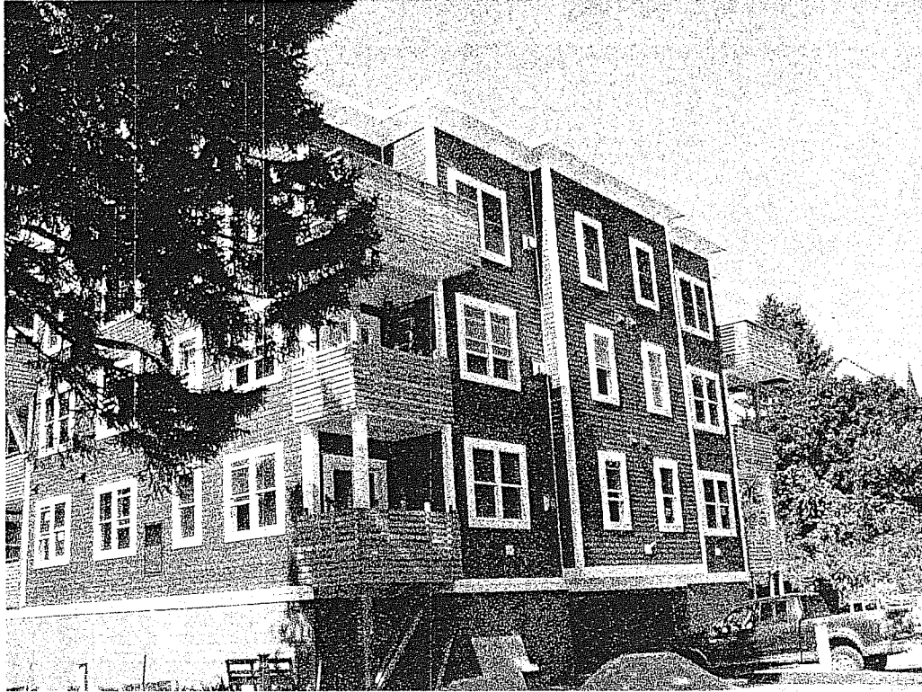
Photo # 1 – Overall view looking at and wall above garage entrance
