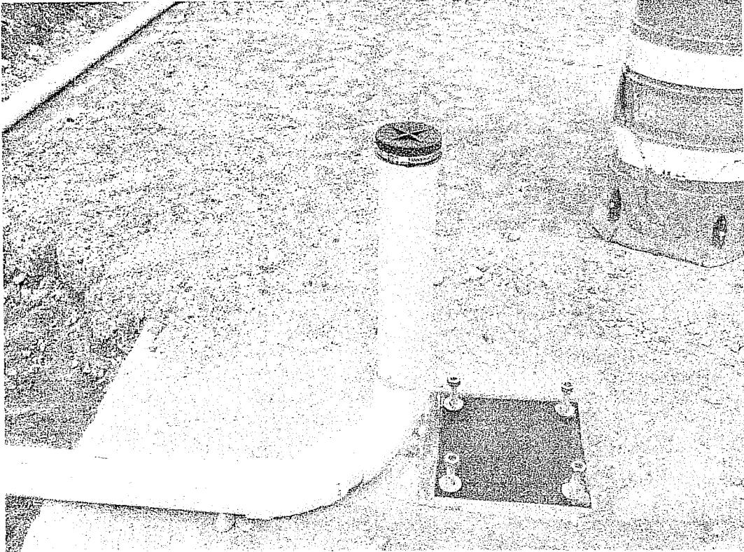
Photo 3 – Sewer pipe adjacent to leveling plate for structural steel column
