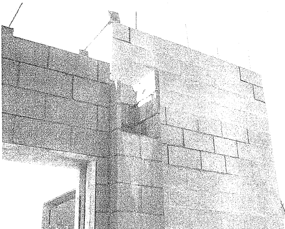
Photo 4 – Beam pocket in masonry near elevator
