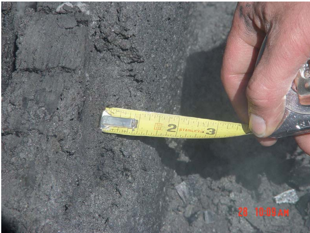
Photograph 14: Measuring the intumescent depth on the side of a joist
