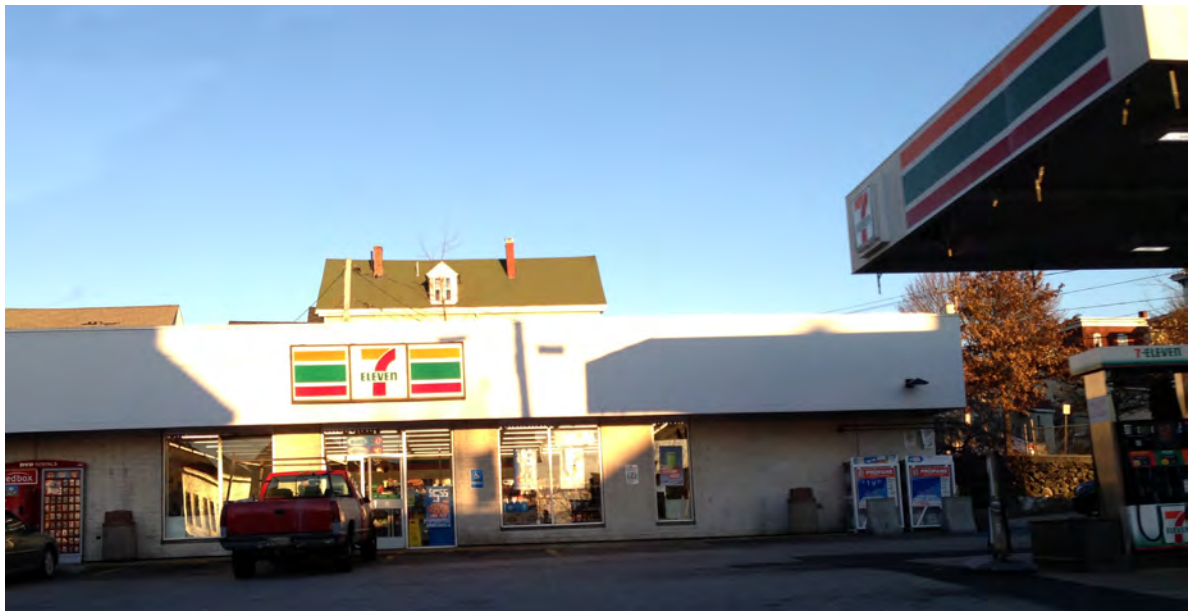
Site viewed from Washington Ave - Existing
