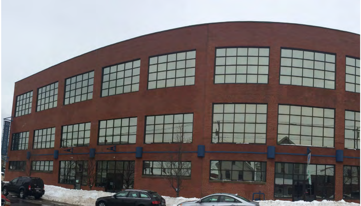
63 Washington Ave. - Red Brick Material Finish
