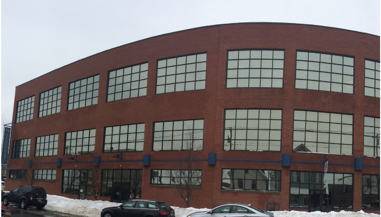
63 Washington Ave. - Red Brick Material Finish
