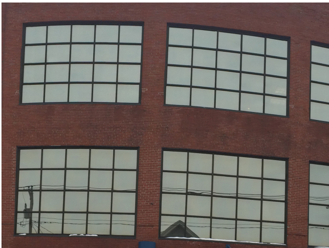
63 Washington Ave. - Fenestration
