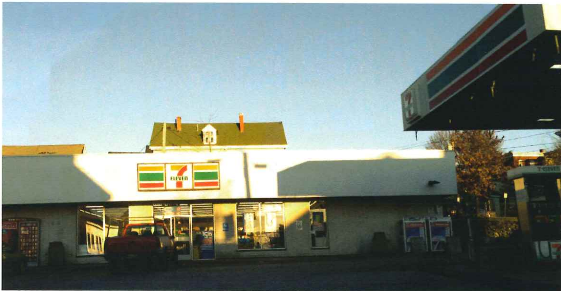
Site viewed from Washington Ave - Existing
