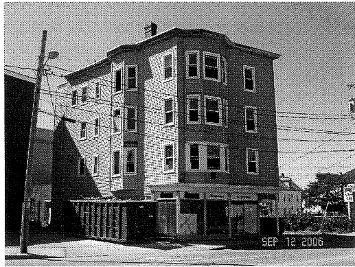
6 Washington Ave – Viewing Southwest
