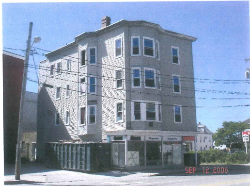
6 Washington Ave – Viewing Southwest
