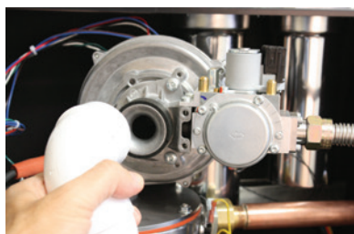
Disconnect combustion air snorkle
