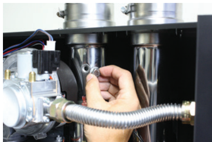
Removing vent stack test port plug
