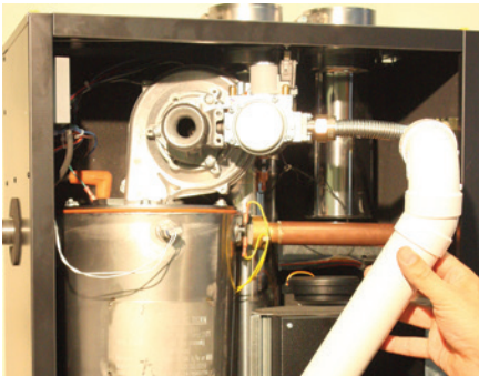
Removing combustion air intake riser
