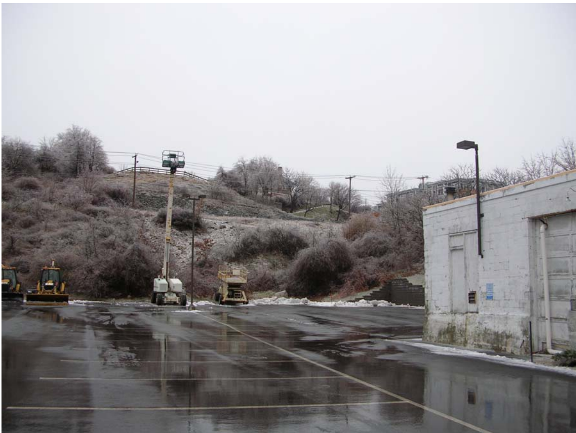
Photo 4: Grade embankment north of Subject Property
