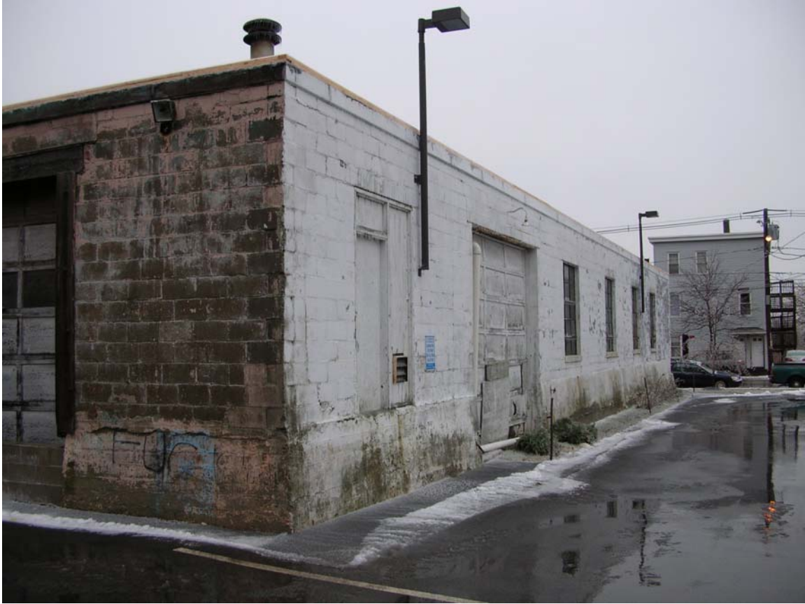
Photo 3: West side of building at 105-107 Washington Avenue
