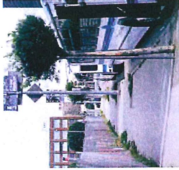
A 7-foot wide sidewalk on a commercial street was widened to 24 feet by extending the sidewalk into the existing roadway to accommodate a double row of trees, a wide walkway and a wide outdoor dining zone.
