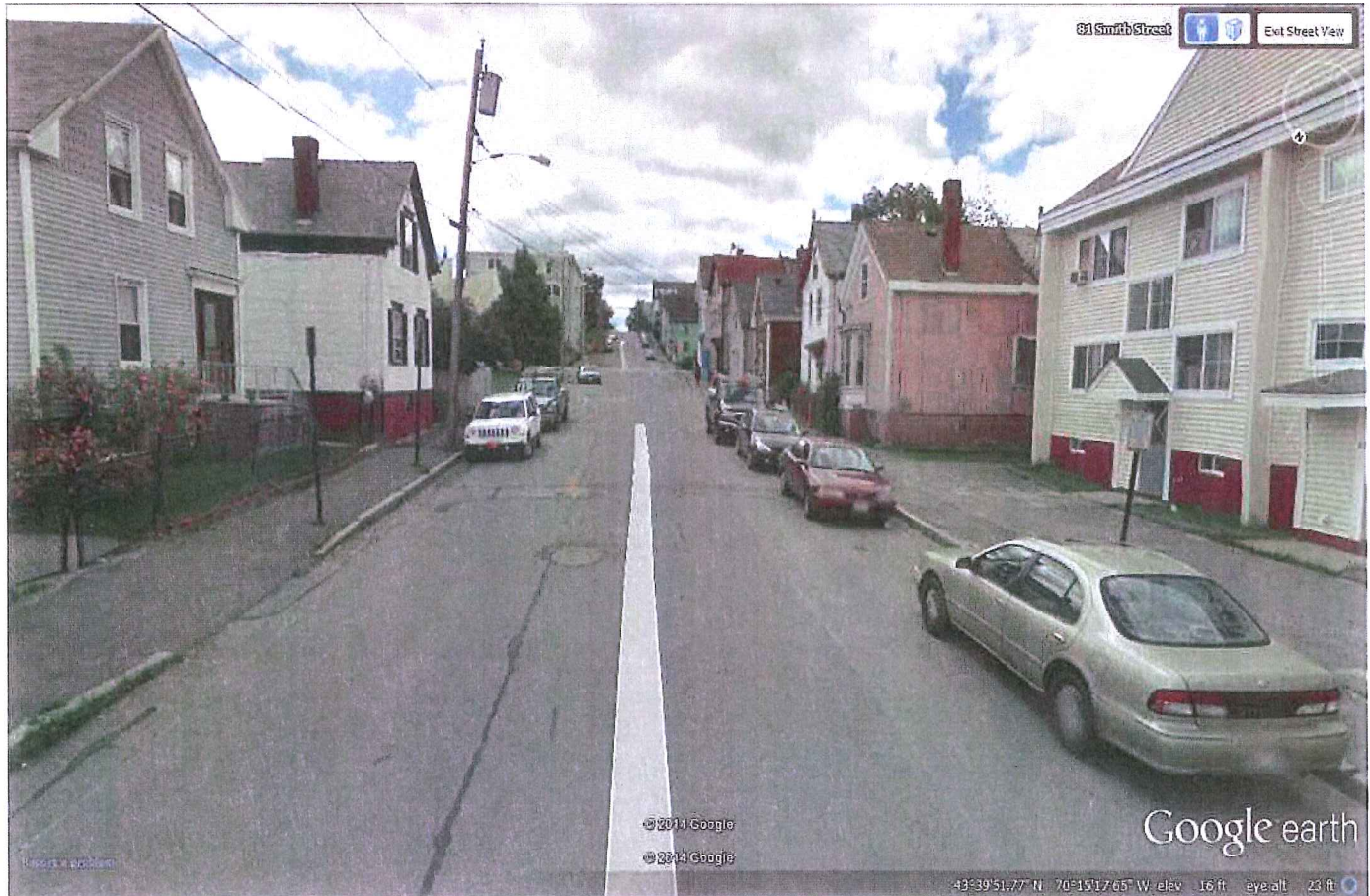
View of Smith Street toward Cumberland Avenue
