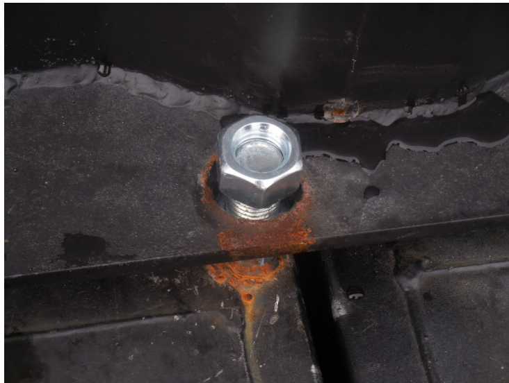
Connection at rear of parapet
