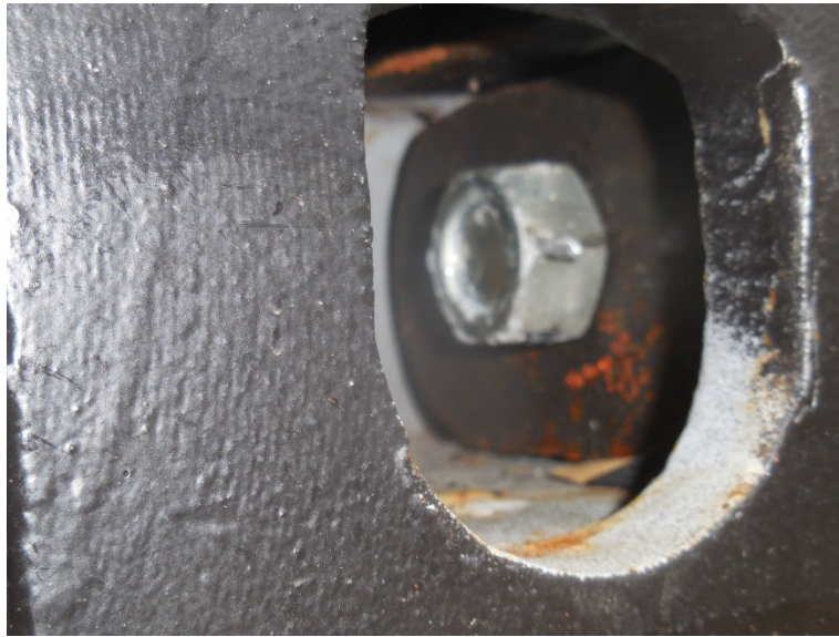
Bolted connection without full nut engagement
