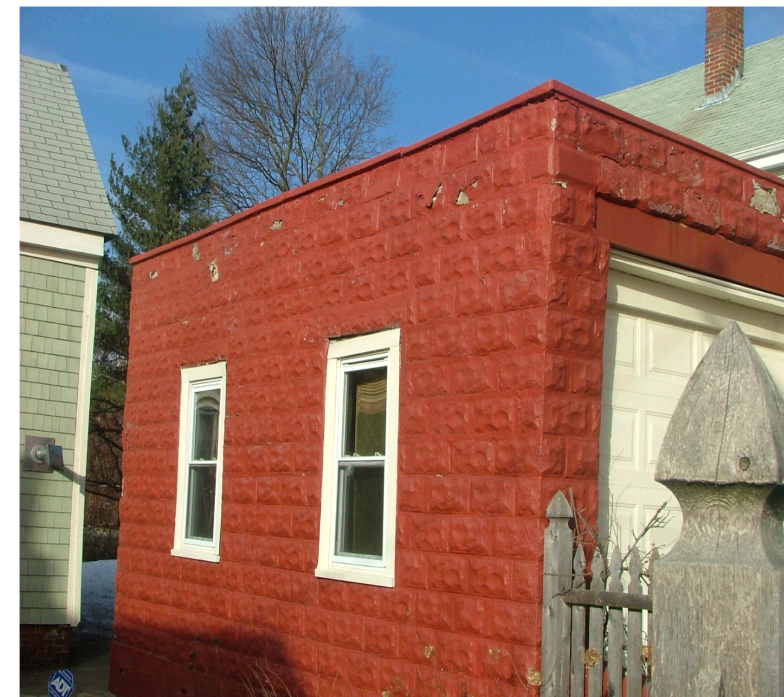
EXISTING GARAG TO BE DEMOLISHED
