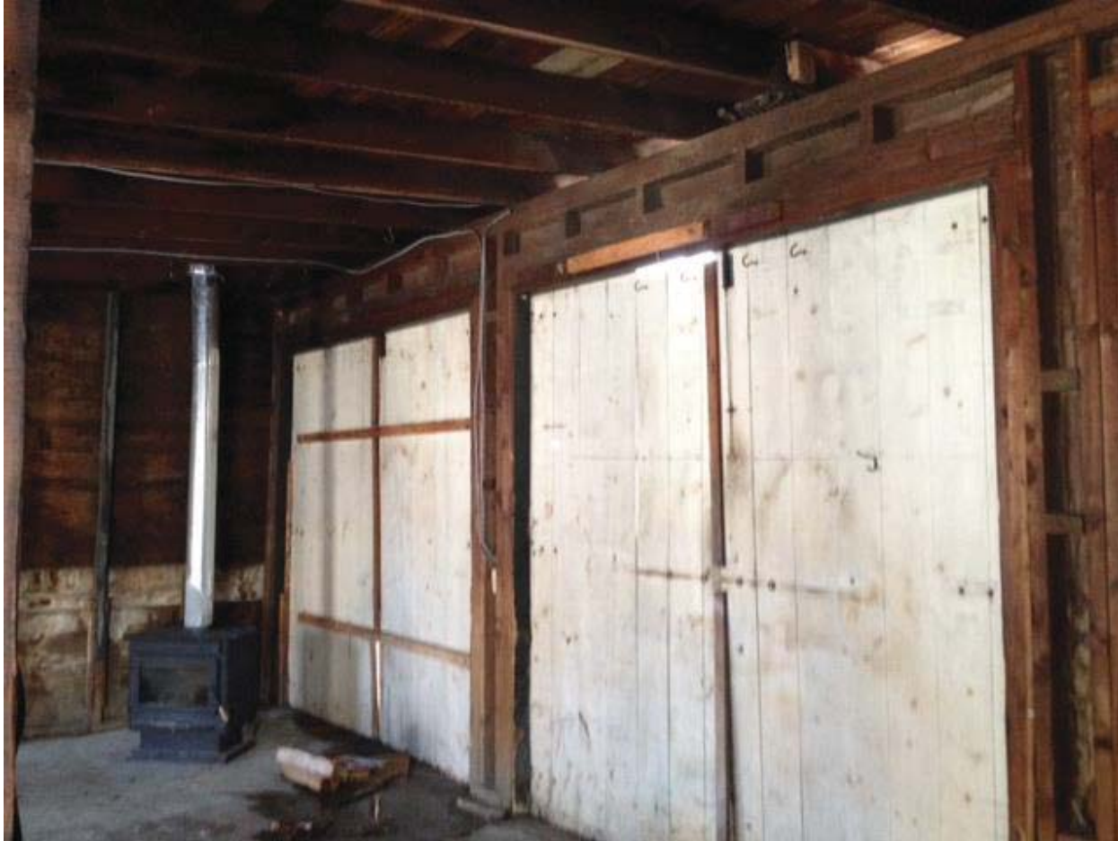
Existing Framing and barn door that will be framed in.
