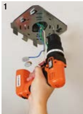
Mount plate to junction box.
