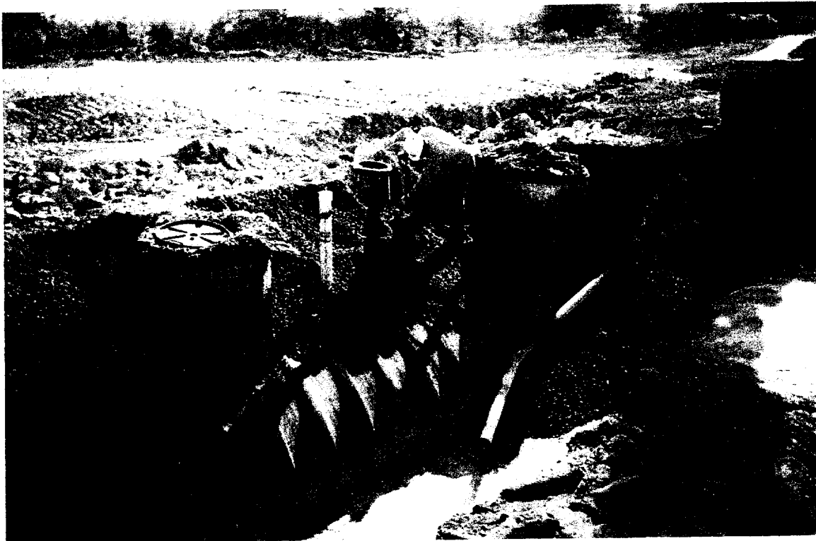
P-2 UST during removal
