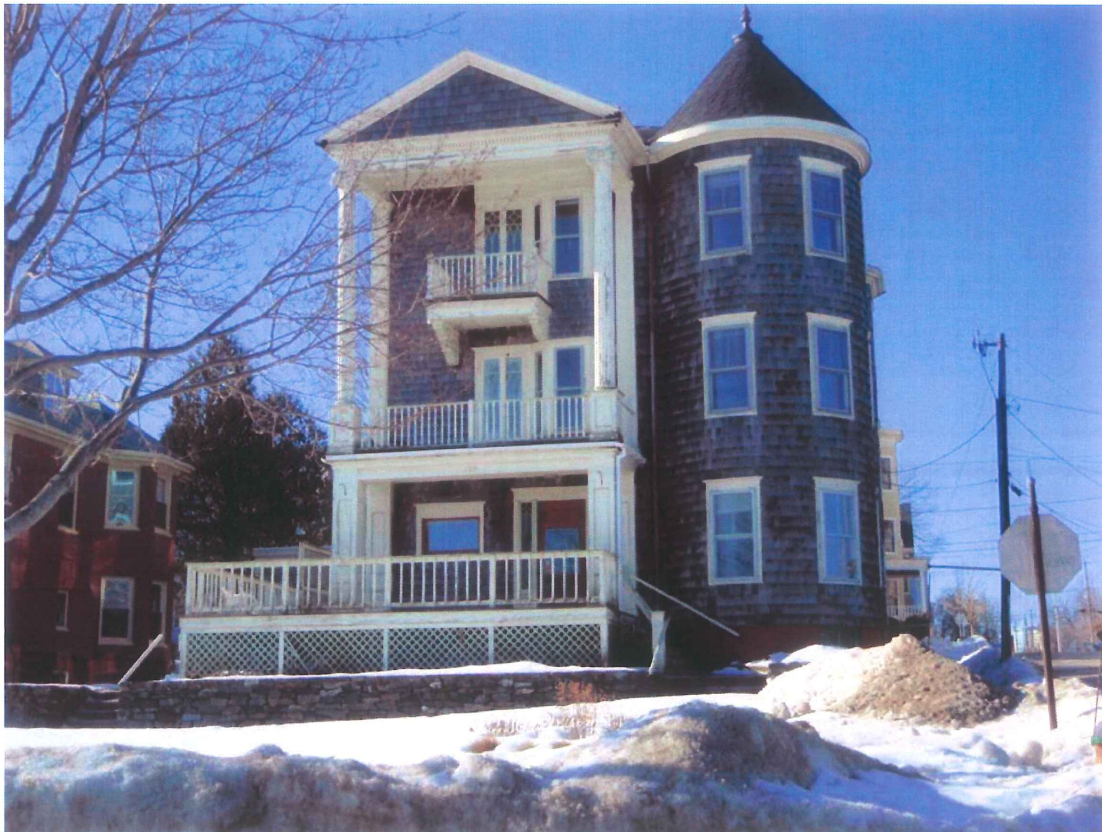
View of existing building from corner of Wilson Street and Eastern Promenade
