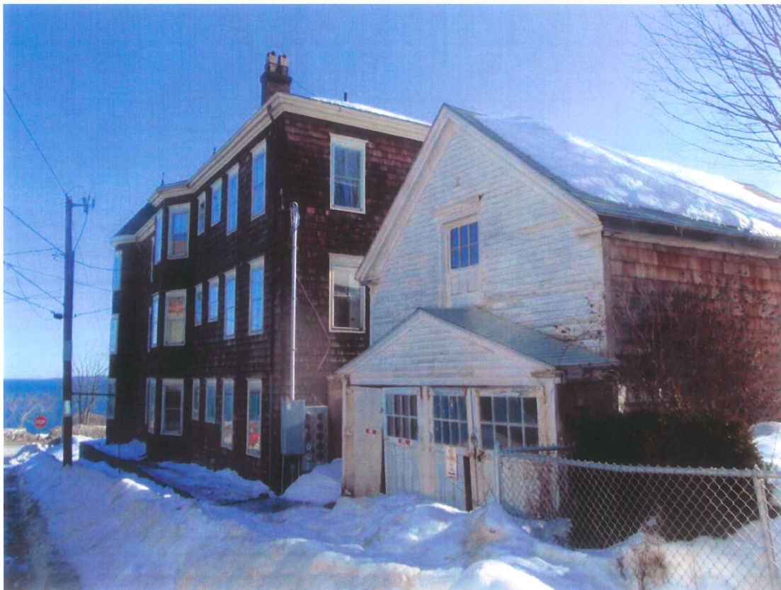
View of Existing Building from Wilson Street
