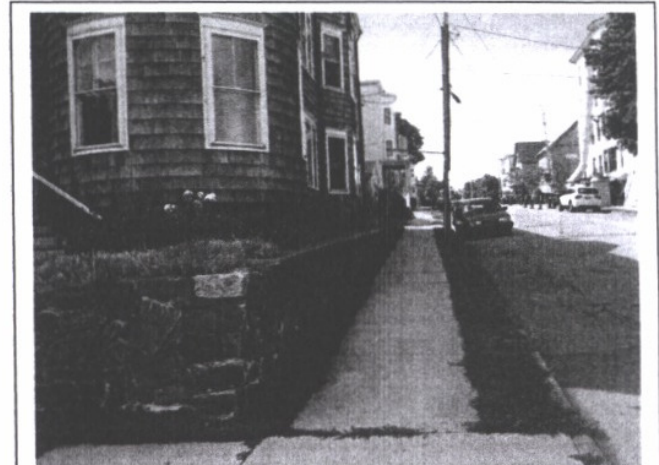
Image 4 - Existing sidewalk on Wilson Street
