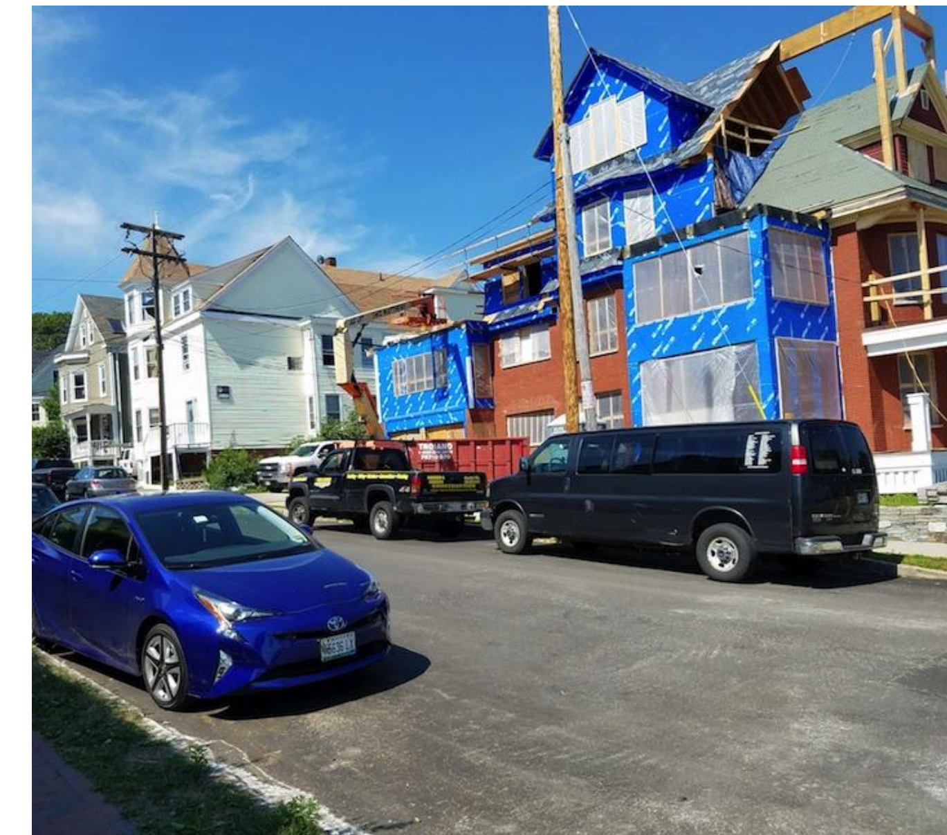
PHOTO FROM CORNER OF MOODY STREET AND EASTERN PROMENADE
